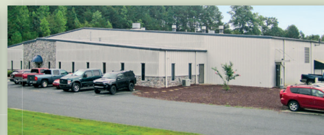
Tower Components, Inc., Ramseur, North Carolina (北卡罗来纳州)
