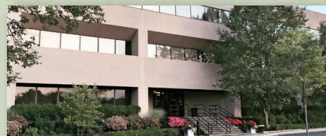
EVAPCO Dry Cooling, Bridgewater, New Jersey (新泽西州)
