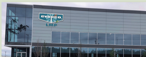
EVAPCO LMP, Laval, Quebec
