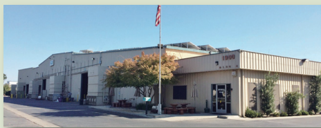
EVAPCO West, Madera, California
