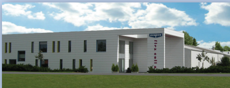
EVAPCO Europe A/S, Aabybro, Denmark
