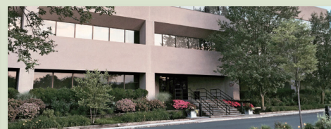
EVAPCO Dry Cooling, Bridgewater, New Jersey
