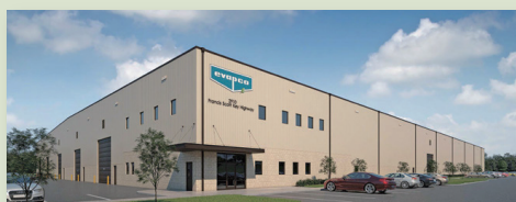
EVAPCO Key Building, Taneytown, Maryland
