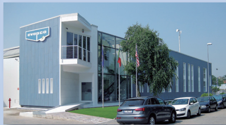
EVAPCO Europe, S.r.l., Milano, Italy
