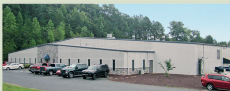
Tower Components, Inc., Ramseur, North Carolina
