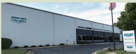
EvapTech, Inc., Edwardsville, Kansas
