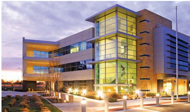
LARGE HVAC APPLICATIONS
