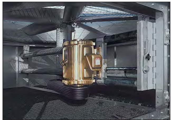
Motor Base Assembly
