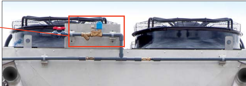
Adiabatic water supply solenoid valve arrangement
