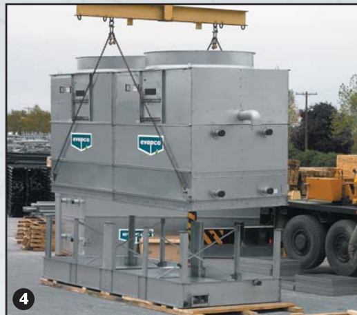
4 Mount Coil/Fan to Basin Section
