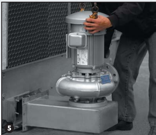
5 Mount Pump and Piping
