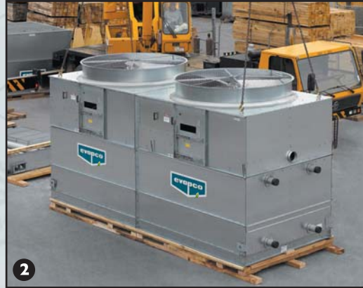
2 Mount Fan Section to Coil Section
