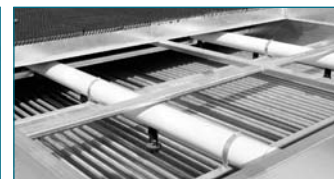
Drift Eliminators Removed for Coil Inspection
