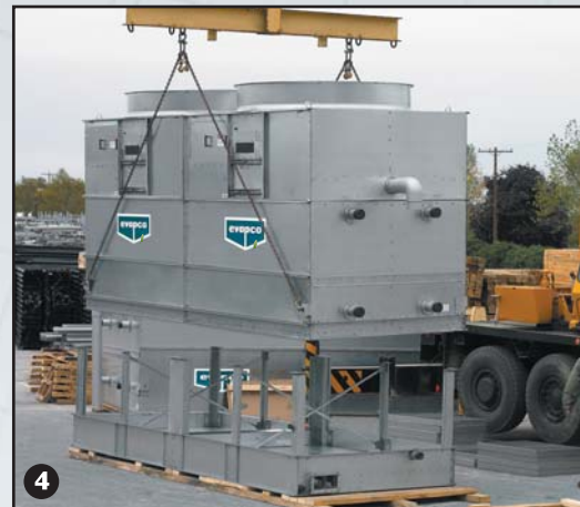
4 Mount Coil/Fan to basin Section
