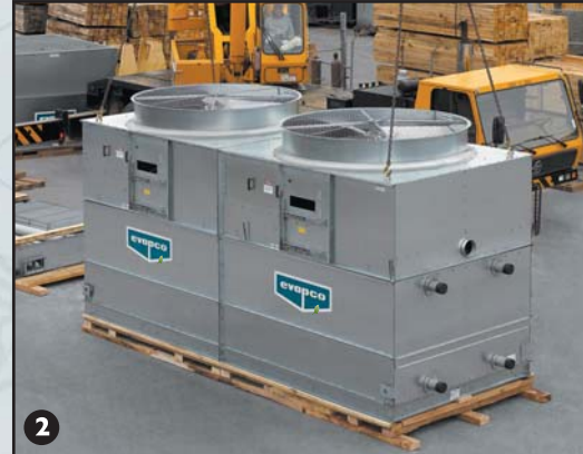
2 Mount Fan Section to Coil Section
