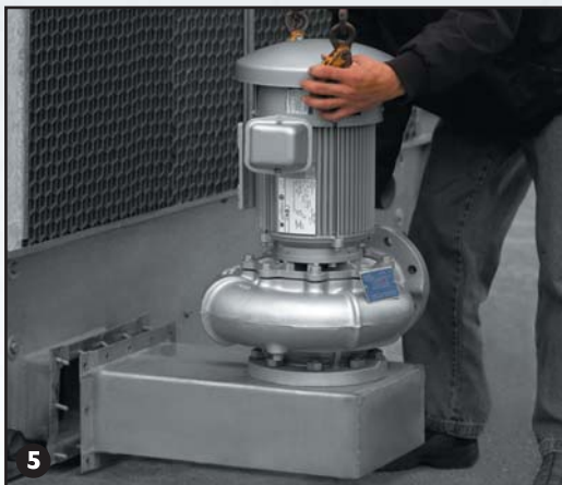
5 Mount Pump and Piping
