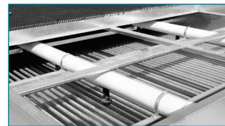
Drift Eliminators Removed for Coil Inspection
